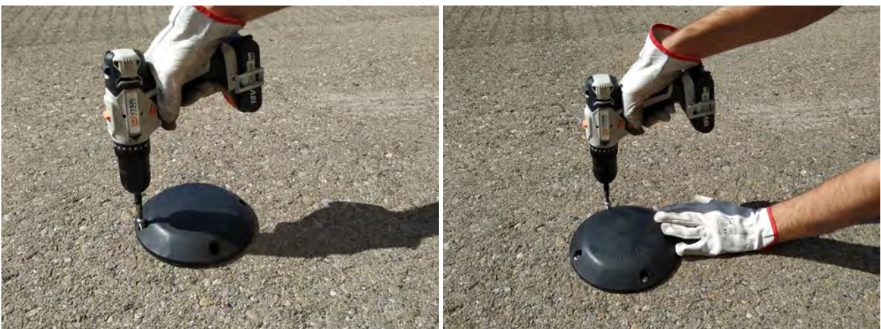
Figure : Screw the node
