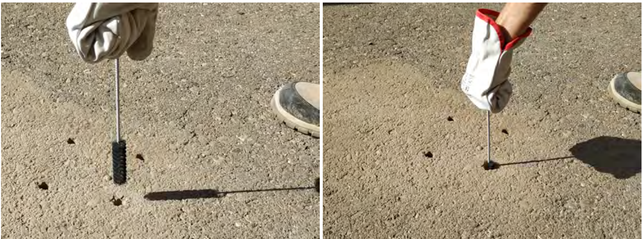
Figure : Brush the hole (step 3)
