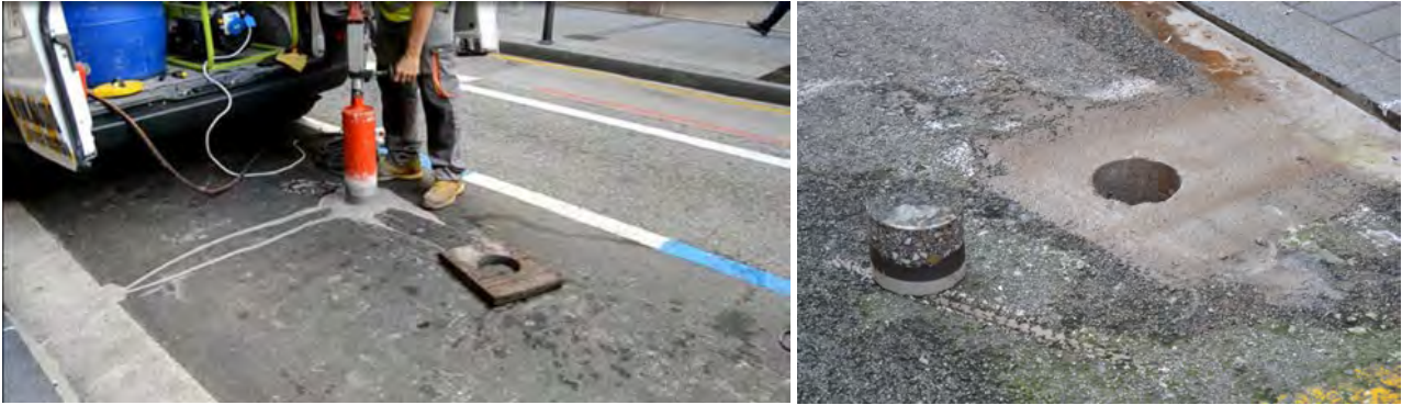
Figure : Making a hole in the pavement
