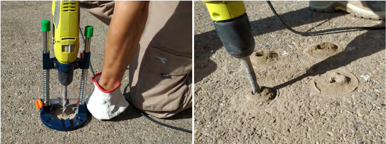
Figure : Drill the holes (step 1)
