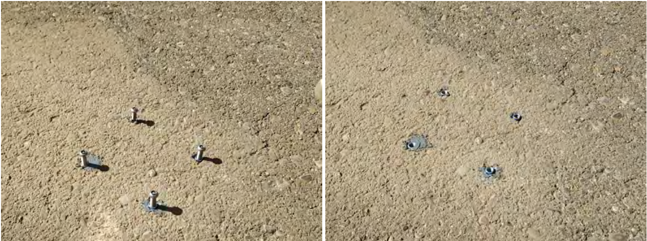
Figure : Final anchor installation (step 7)
