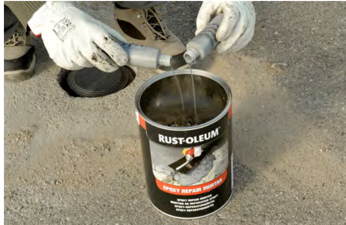
Figure : Pour Epoxy curing agent into the granular resinous material
