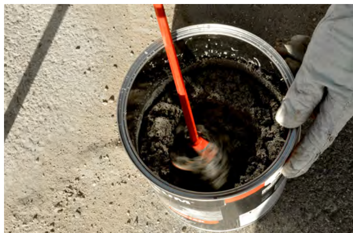
Figure : Pour Epoxy curing agent into the granular resinous material
