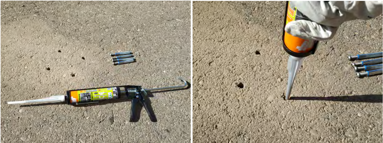
Figure : Inject chemical fixing adhesive (step 5)
